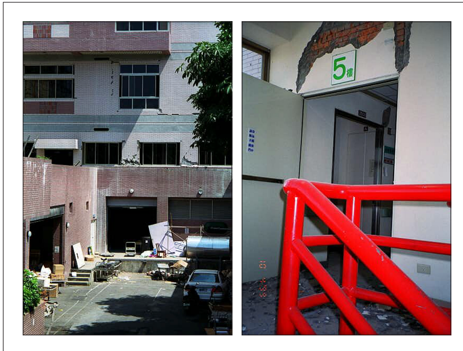
Figure 4-1 The Christian Hospital sustained considerable damage. Photos show (left) part of the exterior damage to the hospital; and (right) interior damage to partitions and ceilings.
