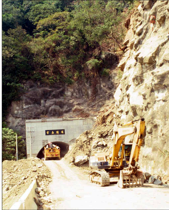
Figure 3-5 Landslide at portal of Yun-Chia Tunnel near Tsao-Ling
