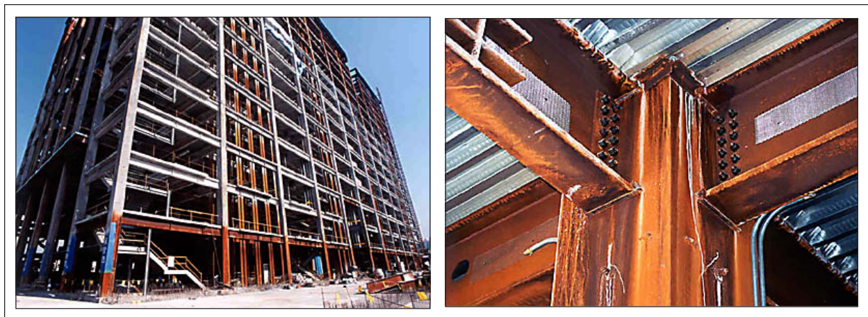
Figure 5-21 14-story steel building under construction with undamaged moment-resisting steel frames
