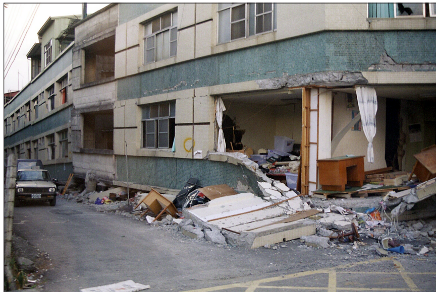
Figure 5-18 Out-of-plane collapse of an infill panel poorly tied to the surrounding frame
