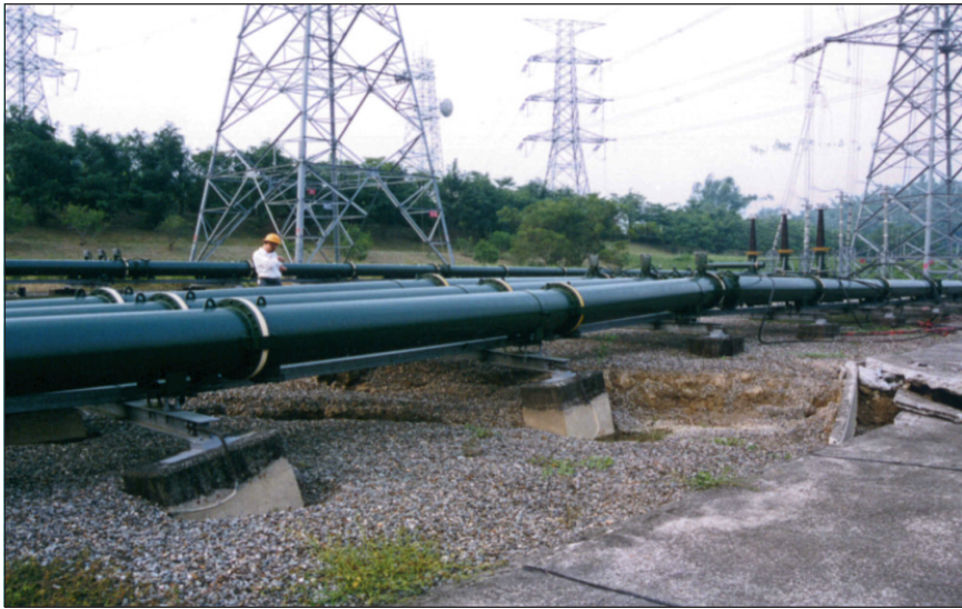
Figure 7-7 Failure of 345 Kv gas insulated line due to liquefaction induced settlement
