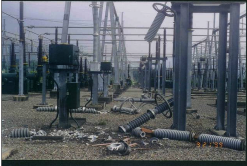
Figure 7-6 Damage at Chung-Liaw switchyard
