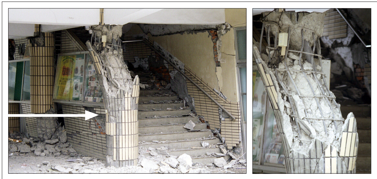
Figure 5-10 Damage to column having widely spaced stirrups and trapped by a partition
