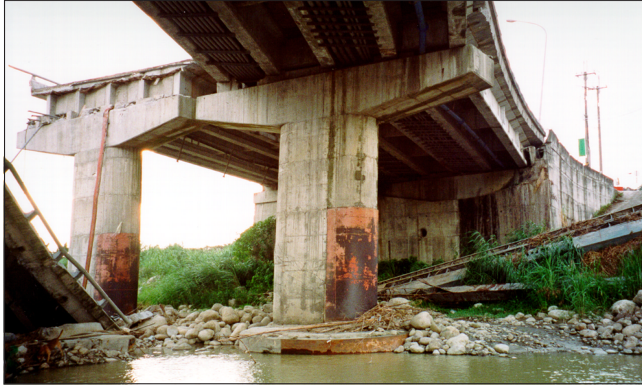
Figure 6-19 Shi-wei bridge showing curvature and skewed alignment of superstructure girders
