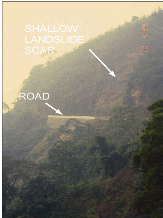
Figure 3-4 Typical shallow landslides intersecting a mountain road
