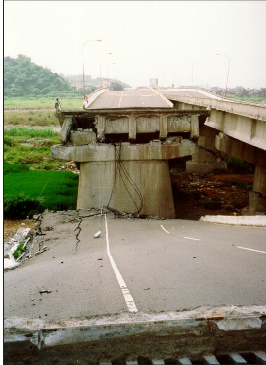
Figure 6-11 Collapsed span in the Wu-shi bridge (east)
