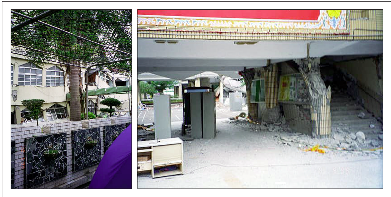
Figure 4-7 Typical damage to schools due to short-column effect and eccentricity
