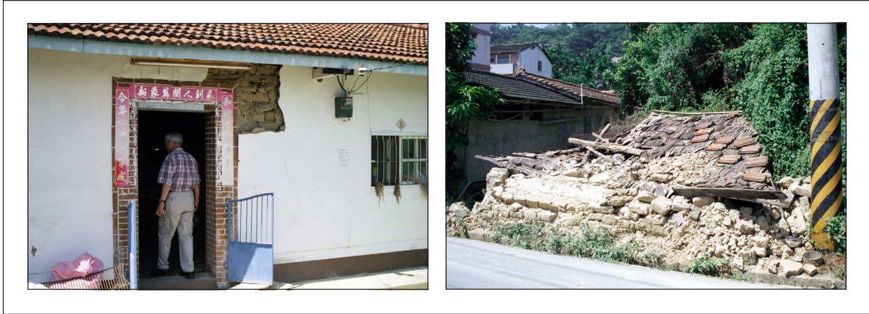
Figure 5-25 Cosmetic damage (left) and complete collapse (right) of unreinforced masonry structures located 15 feet apart
