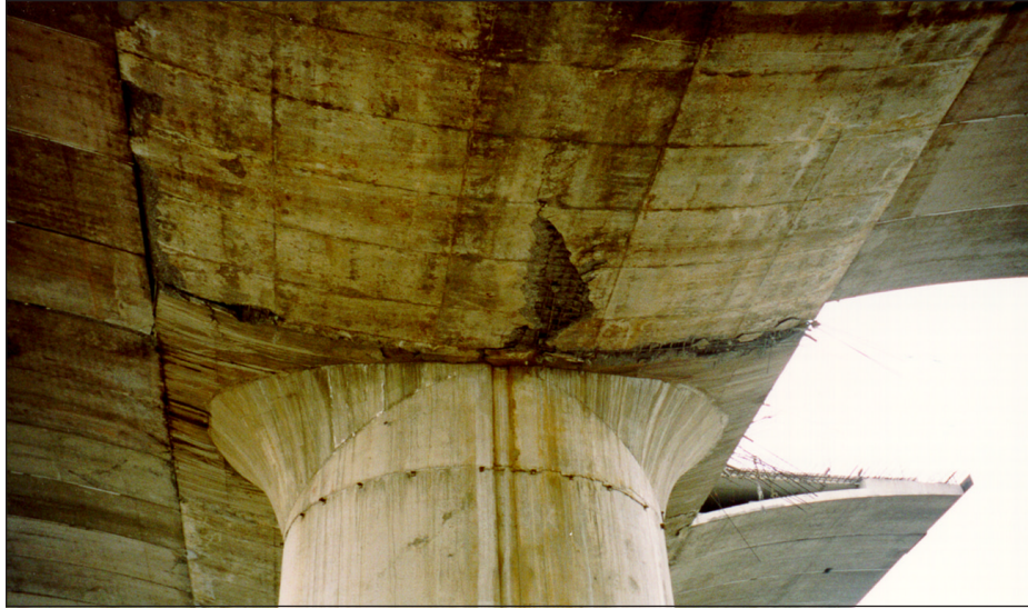
Figure 6-22 Damage to the soffit of the main girder near the pylon of the Ji-lu bridge; missing cantilevered section (right) had not been placed at time of the earthquake
