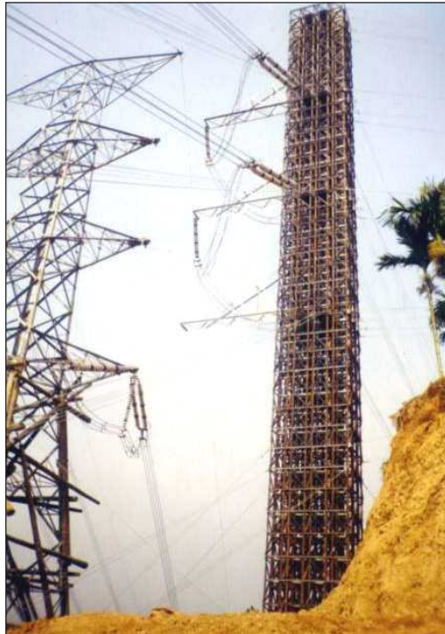
Figure 7-5 Failed transmission tower replaced by a temporary tower
