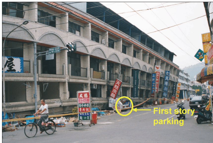
Figure 5-5 Soft-story failure of building having numerous large openings at first story on street side
