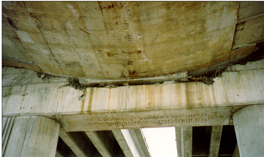
Figure 6-23 Pounding damage and shear cracks in the bent cap of the north abutment of the Ji-lu bridge
