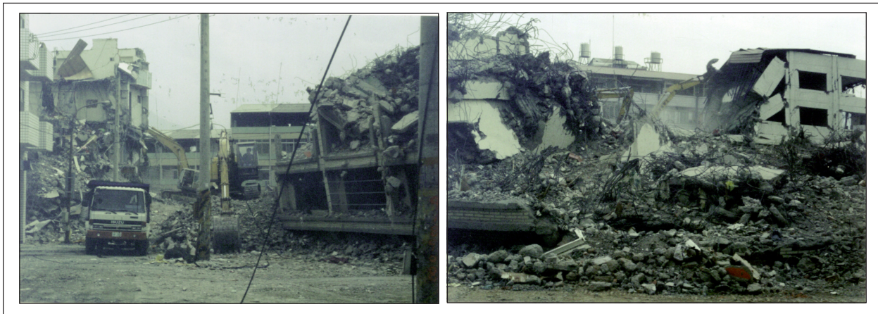
Figure 10-6 Demolition of severely damaged multi-family apartment complex
