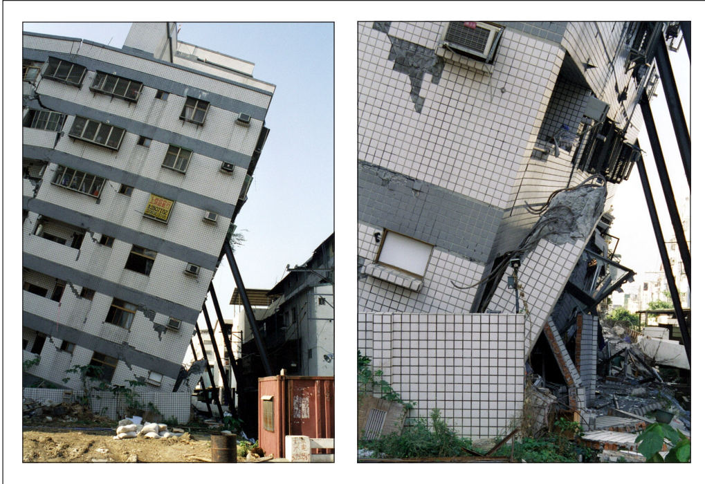
Figure 5-20 Collapse due to poor detailing practice
