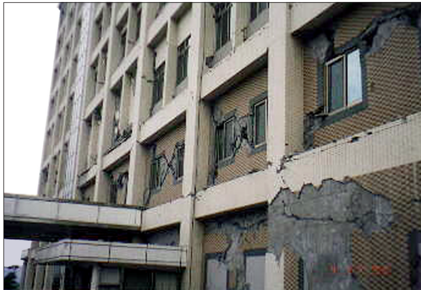
Figure 4-6 Damage to an exterior wall of the Shiu-Tuan Hospital in Nantou county
