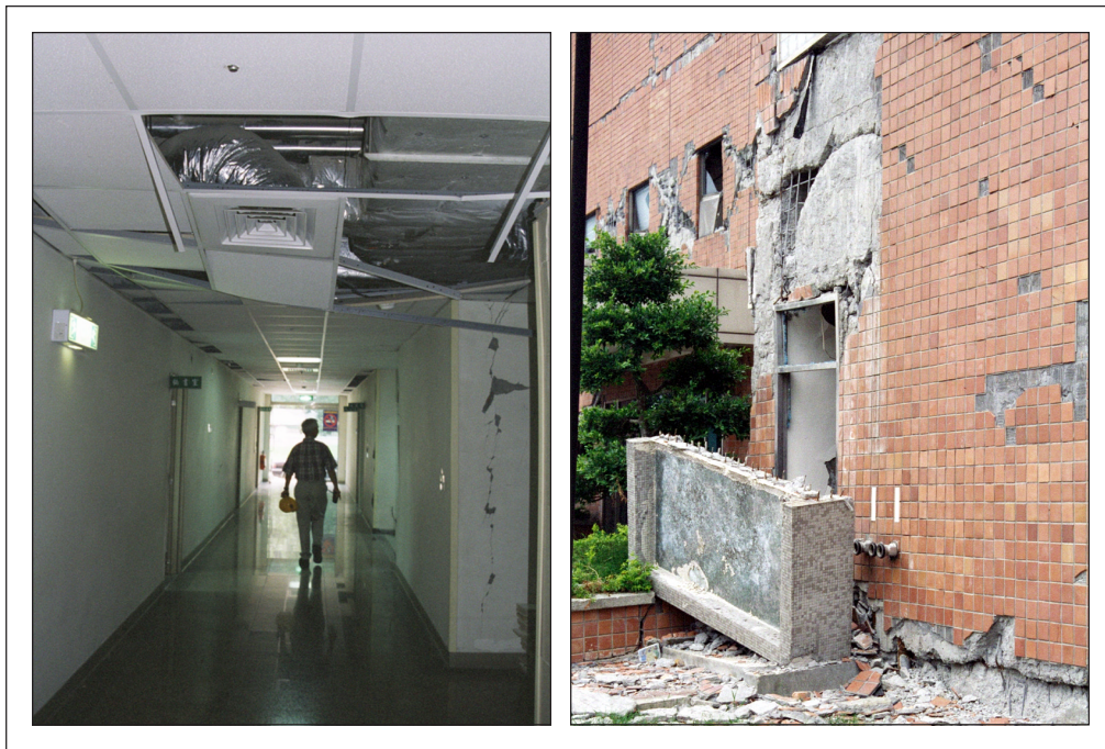
Figure 5-24 Examples of interior and exterior nonstructural damage that may prevent safe egress; collapse of suspended ceiling (left) and collapse of canopy above an exit door (right)
