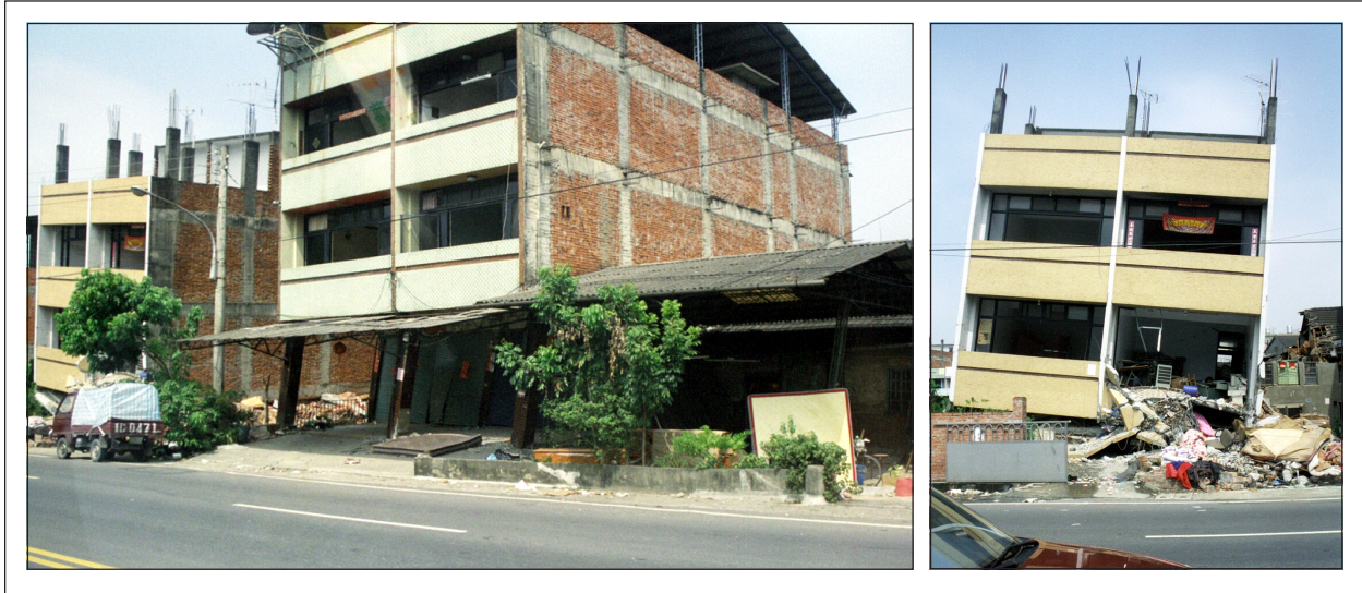
Figure 5-4 Large sway in progression toward collapse (left) and building failure due to soft first story (right)
