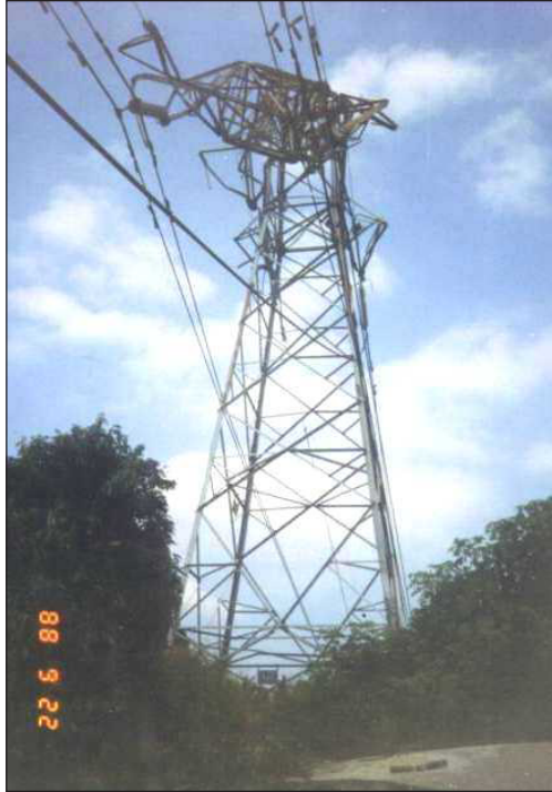
Figure 7-4 Transmission tower with top portion collapsed
