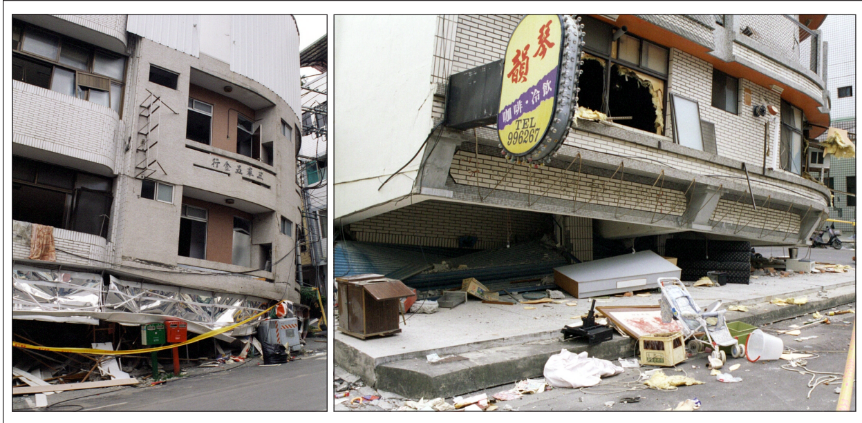
Figure 5-8 Buildings located on street corners toppled toward the intersection as a result of soft-story damage
