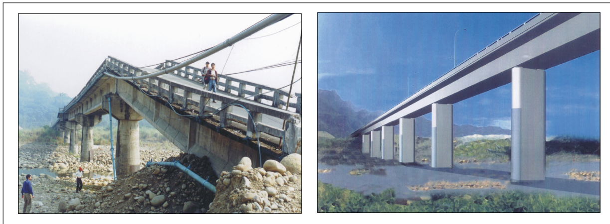
Figure 6-27 Long-men Bridge after earthquake (left) and after reconstruction (right)
