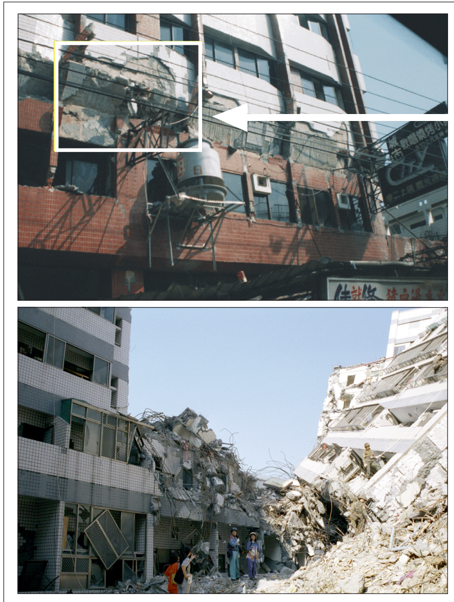
Figure 5-19 Severely damaged building complex; (top) out-of-plane collapse of third story infill wall; (bottom) collapse due to poor detailing practice
