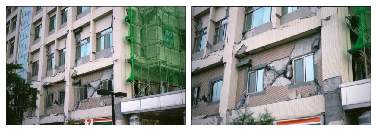
Figure 5-17 Hospital with severe damage to nonstructural infill walls but minor (cosmetic) damage to structural elements
