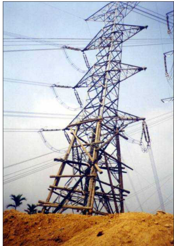
Figure 7-1 Transmission tower tilted and deformed
