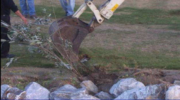
CONSTRUCTION-Fullerton Golf Course, CA, Derrick 11-20-2007
