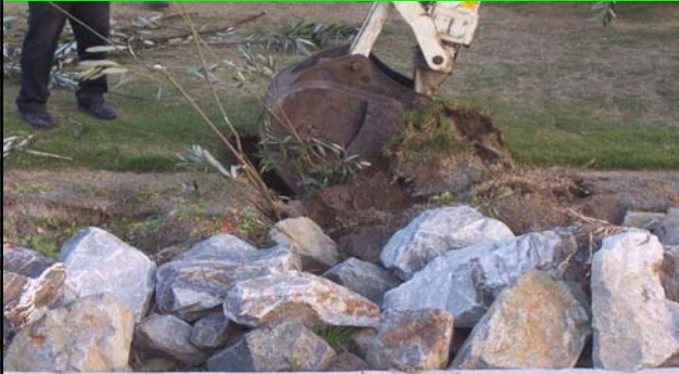
CONSTRUCTION-Fullerton Golf Course, CA, Derrick 11-20-2007
