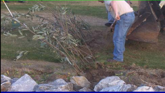
CONSTRUCTION-Fullerton Golf Course, CA. Derrick 11-20-2007
