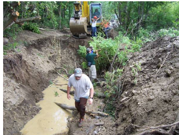
McKinstry Creek during construction July 2005
