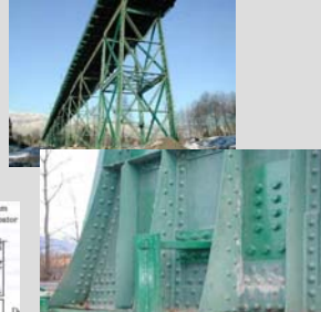
Lions Gate Bridge North Approach
