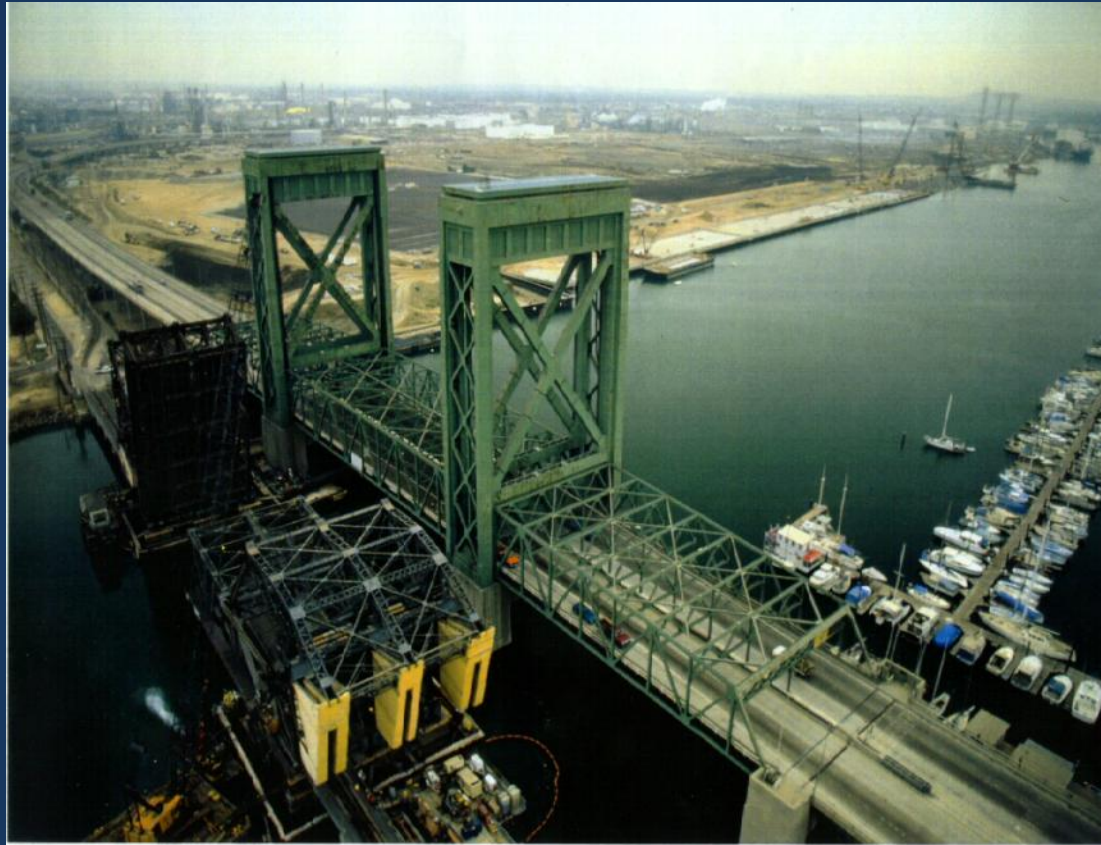
Schuyler Heim Bridge, Long Beach CA Martin Marietta Composites
