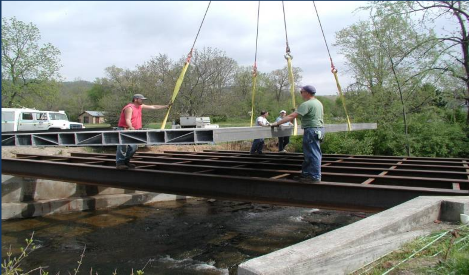
LaChein Bridge Monroe, WV 2002 Bedford Reinforced Plastics
